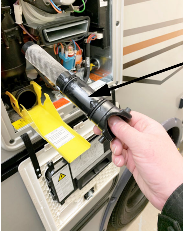
Water inlet strainer pulled out and removed. -Typical View
